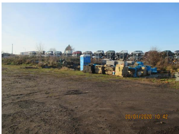
View of site facing south west
